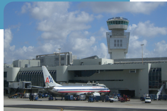
Miami International Airport, one of North America's largest international hubs, uses Stormceptors on its runways.
